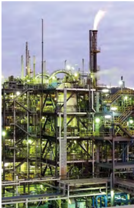
Orica's world-scale cyanide manufacturing facility is located in Yarwun, Australia.
